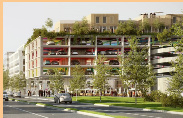
Image source: Brisac Gonzalez ( http://www.brisacgonzalez.com/parking-plus )
