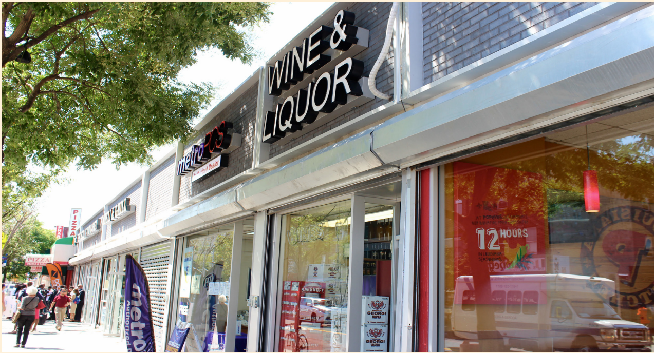
Improved storefronts funded by SBS. Sutphin Boulevard, Queens.
