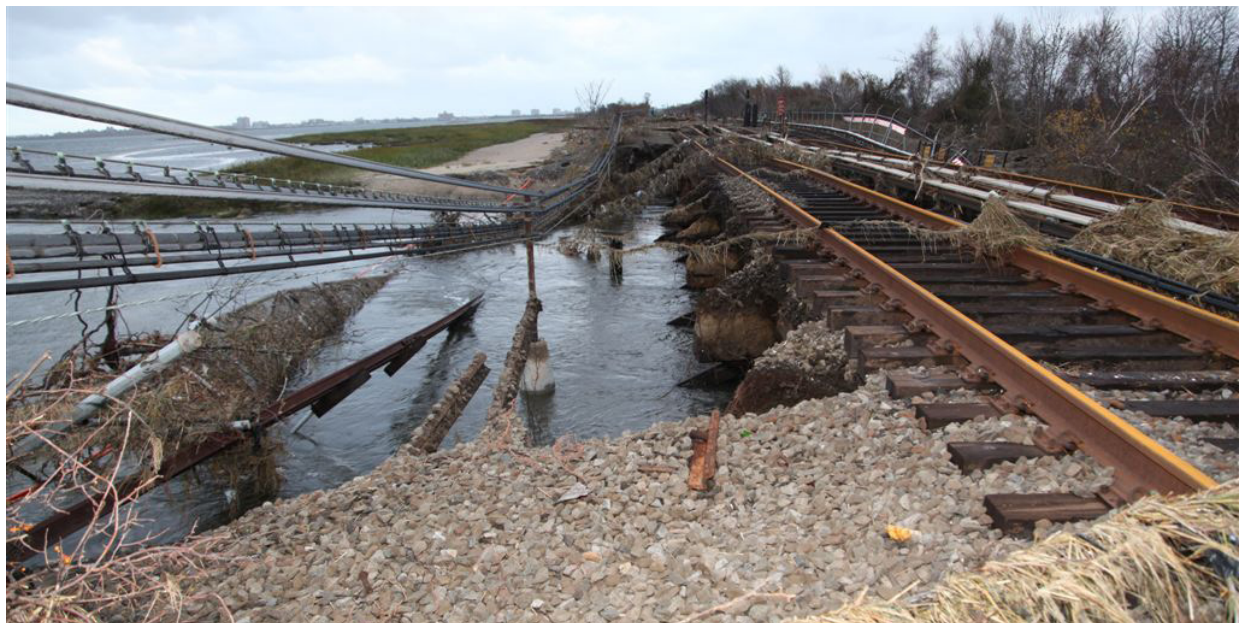
Hurricane Sandy damage on the New York City Subway's Rockaway Line (A train). Source: MTA (flickr: https://flickr.kr/p/dpxEmN )
