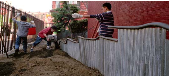
MS 131 Students back-fill soil around new corrugated steel "water element"
